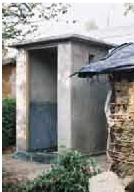
New toilets - doors to come!
